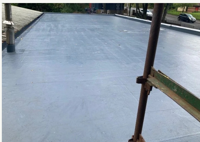
AFTER / LIQUID-WATERPROOFING FINISH
